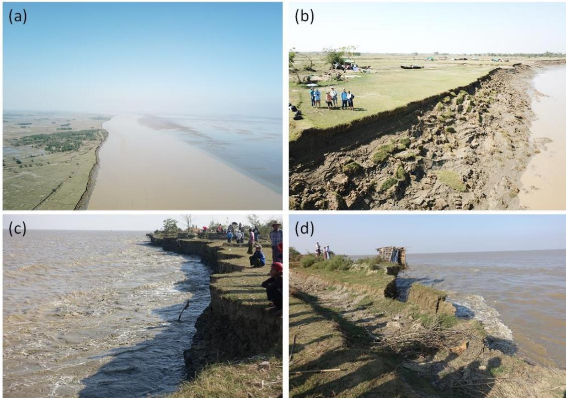
Figure 2.10 (a) The stream channel near the bank line at Mamauk (the UAV camera focussing towards upstream), (b) The side slope of erodible bank composed of very fine (clay type) materials (picture taken before the tidal bore came), (c) After the passage of tidal bore, strong tidal currents take place causing severe bank erosion and (d) Occurrence of bank collapse owing to base erosion resulting from strong currents following the passage of bore front
